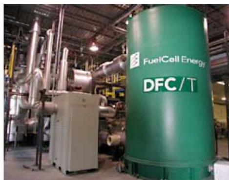
FCE's Direct FuelCell® Hybrid model, a MCFC system with a gas turbine (www.fce.com)
