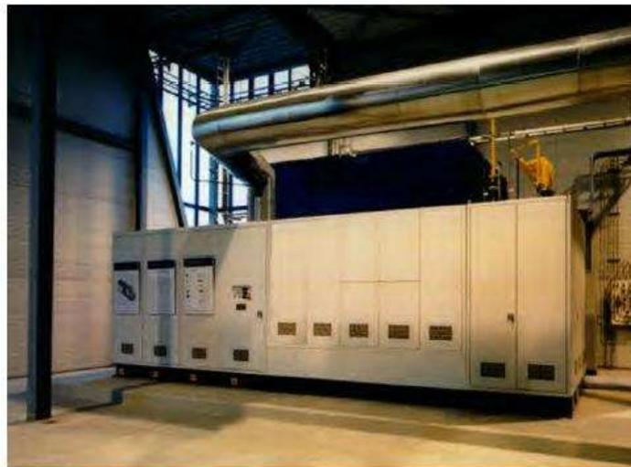
Siemens Westinghouse tubular solid oxide fuel cell
